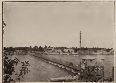
MAUDE BRIDGE ACROSS THE TIGRIS RIVER AT BAGHDAD
